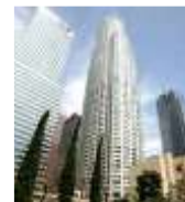
U.S. Bank Tower, Los Angeles (100% stake)
