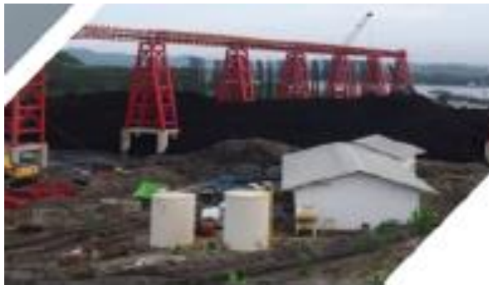
MOGL – CB7 – Oil and Gas Unit
