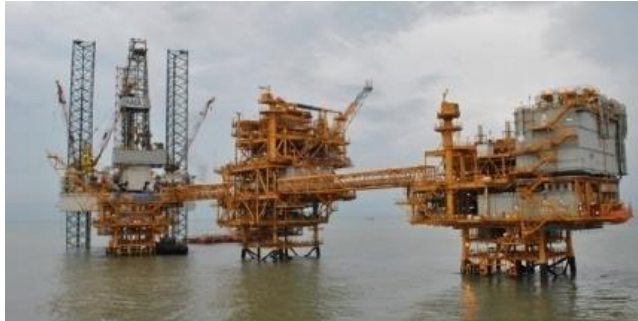
Daman Development Project (ONGC), India. Completed 1Q2016
