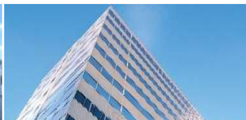
Omori Prime Building, Tokyo, Japan
