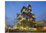
Keppel Merlimau Cogen Plant (KMC)
