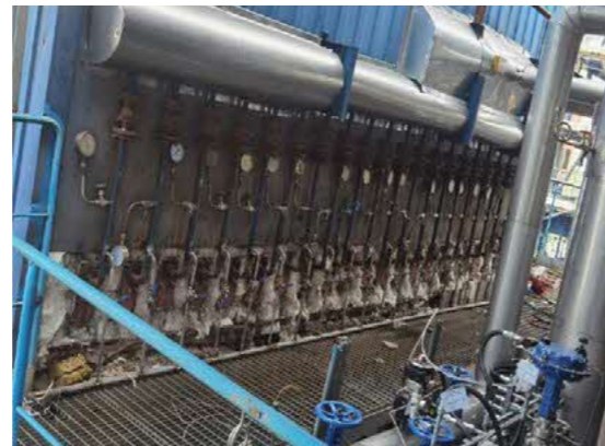
Upgrades to Ammonia Liquid Vaporisation System in Denitrification Furnace
