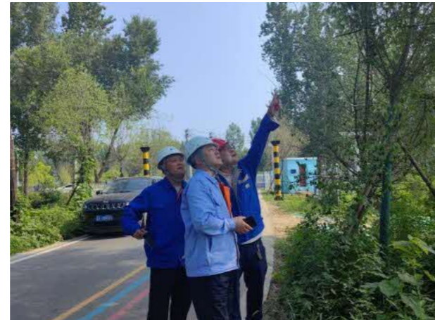
Engineers Are Conducting Safety Inspection of Heating Networks
