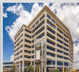
VILLAGE CENTER STATION I Denver, Colorado
