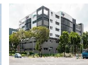
30 Marsiling Industrial Estate Road 8
