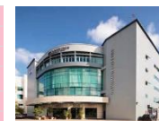
25 Changi South Ave 2
