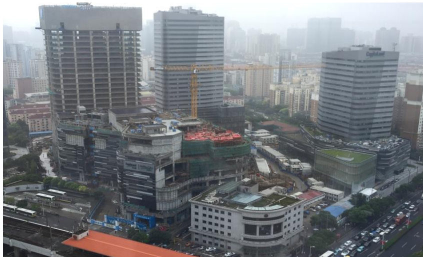
Overall Construction On Track
