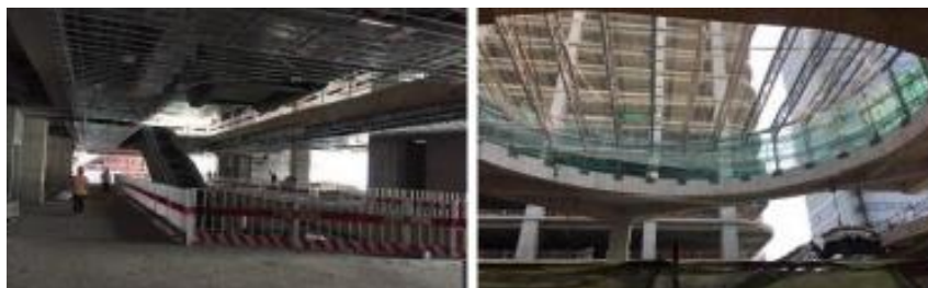
Interior Fitting Out In Progress
