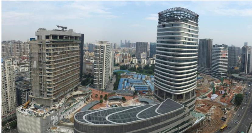
Overall Construction On Track
