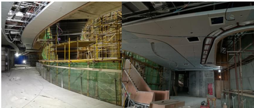
Interior Fitting Out In Progress
