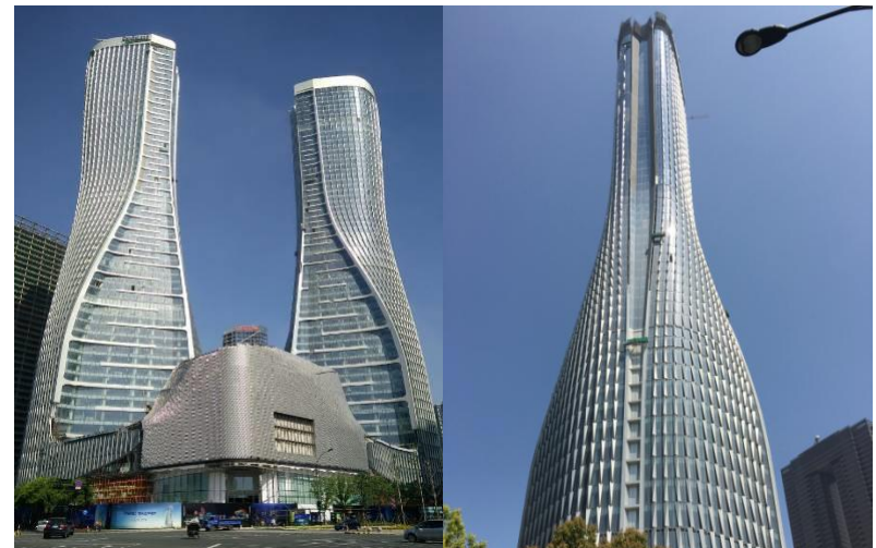
Façade Is Completed
