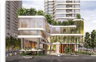
Yanlord Century Mansion, Shenzhen 仁恒世纪大厦, 深圳
