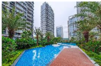
Yanlord North Shore Gardens, Zhuhai 仁恒北岸苑, 珠海
