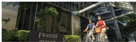
Frasers Tower, Singapore
