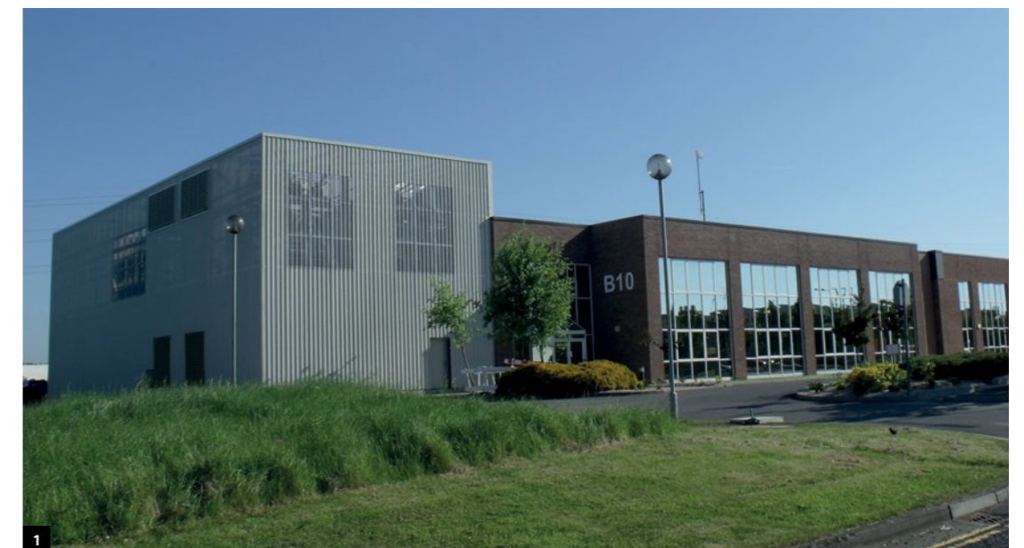
1. The REIT acquired its second data centre asset in Dublin, Keppel DC Dublin 2 (formerly B10 Data Centre).
