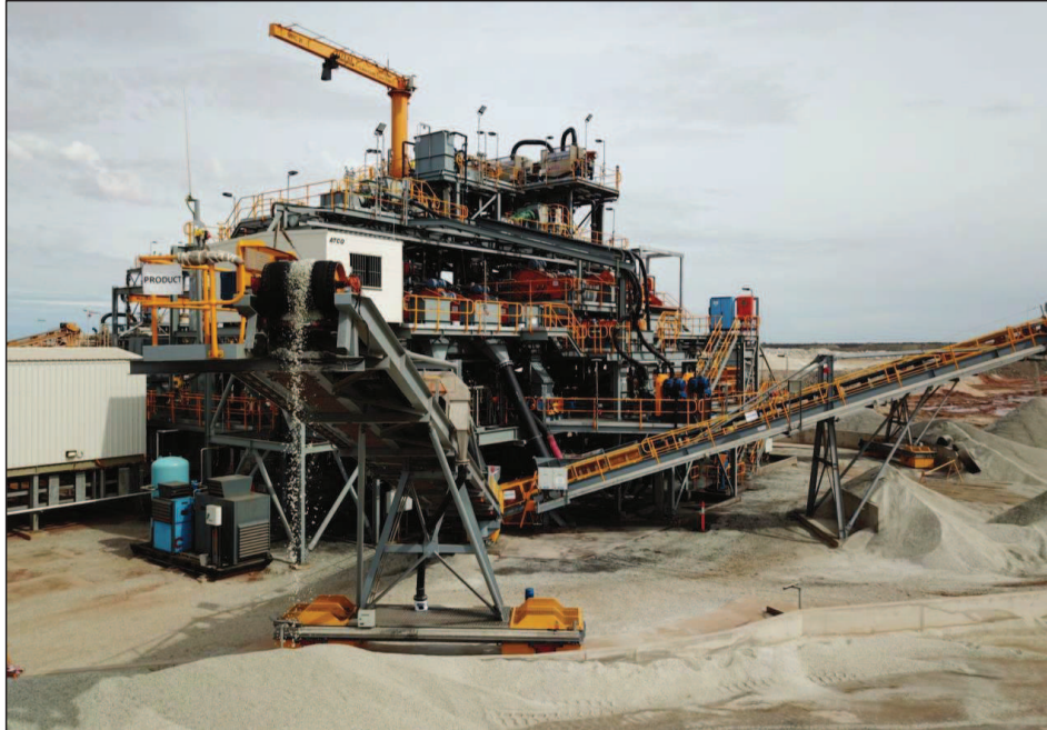
Figure 20: Stage 1 DMS plant
