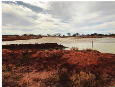
Tailings discharge into Boreline Pit
