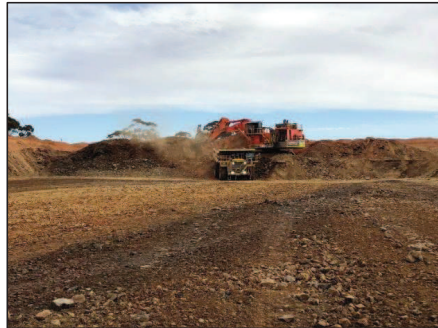
Mining excavations to provide additional sump capacity
