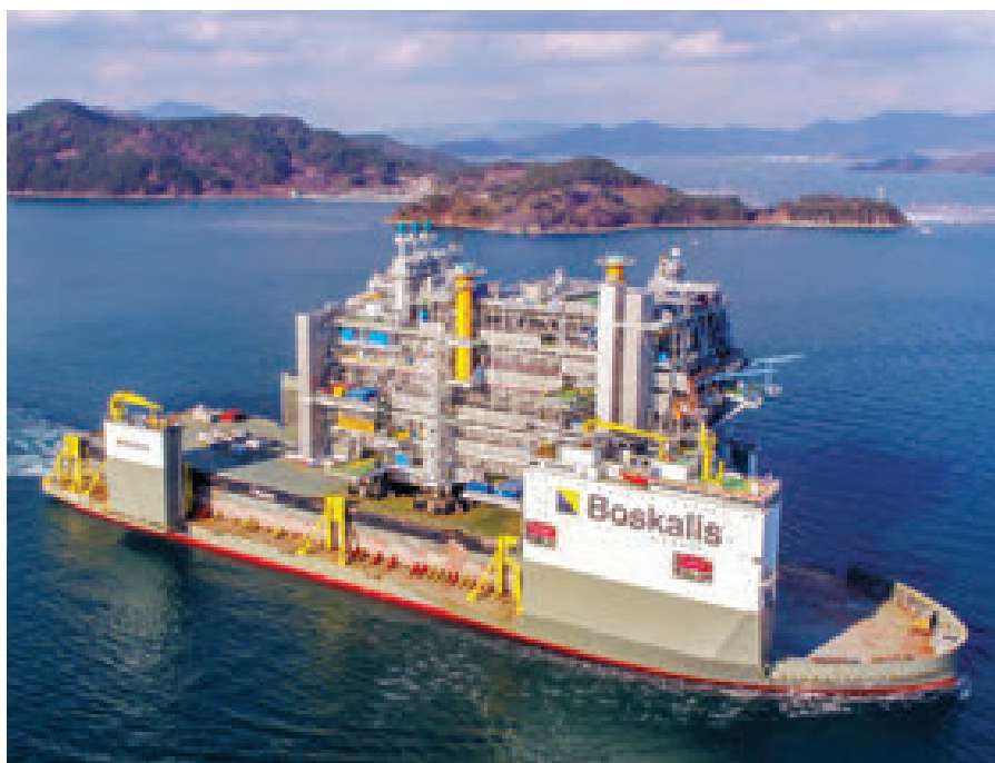
Hot oil heaters integrated onto offshore platform enroute to destination, Norway
