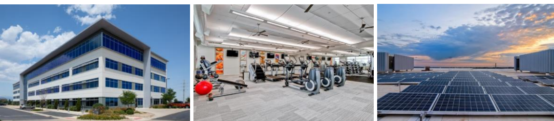
From left to right: 105 Edgeview's building exterior, fitness centre and solar panels atop the building.
