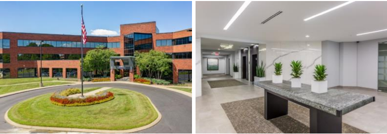
From left to right: Bridge Crossing's building exterior and its expansive and modern lobby.
