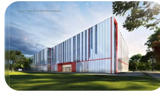
GDS Nusajaya Tech Park Data Centre Campus Fire protection for Blocks A, B and C with 69.5 MW Phase 1 campus
