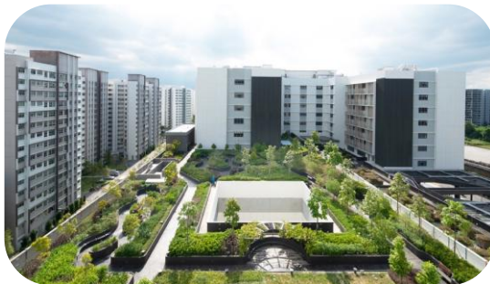
Sengkang General Hospital Installed all fire protection systems including sprinkler, alarm, hydrant and clean gas
