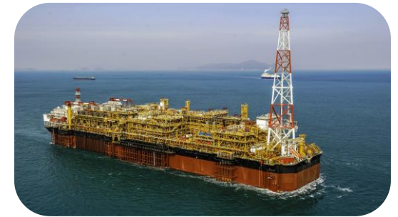
Shell Gato do Mato FPSO Integrated fire and gas detection, suppression and control systems
