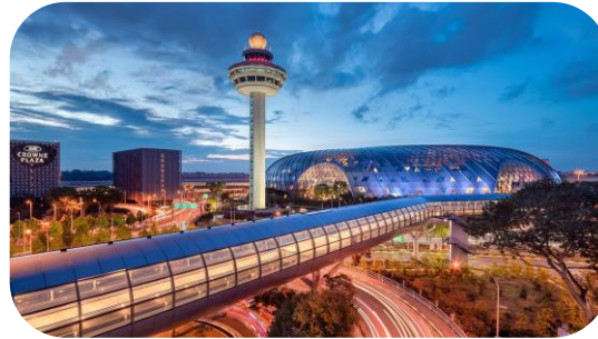
Changi Airport Terminals 1 and 2 Fire protection works across airport terminal infrastructure
