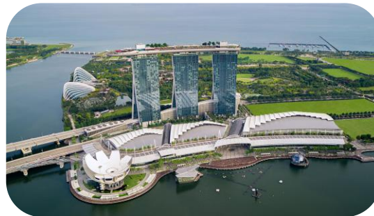
Marina Bay Sands Integrated Resort Fire protection installation
