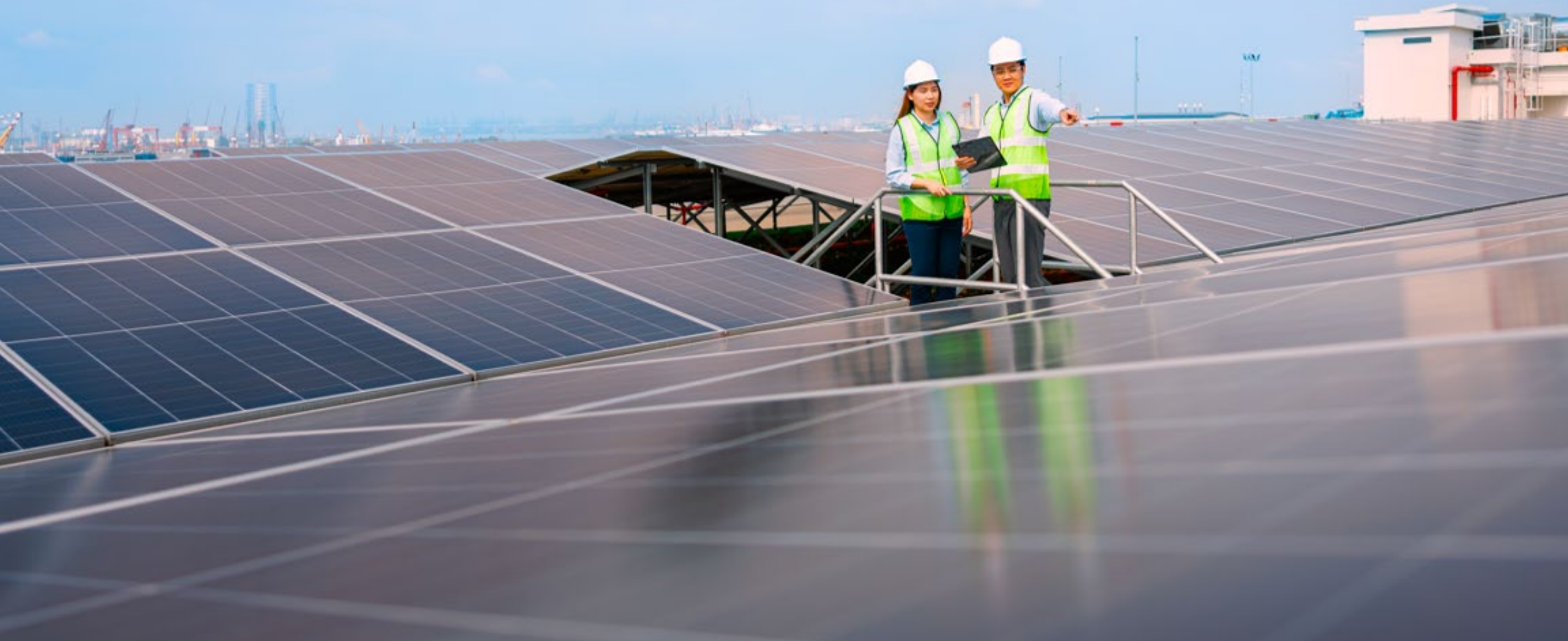
Rooftop solar panels at Mapletree Joo Koon Logistics Hub, Singapore
