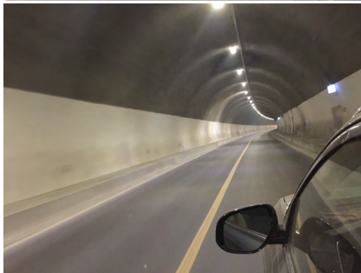
Photo 1. Mine Haulage Road
