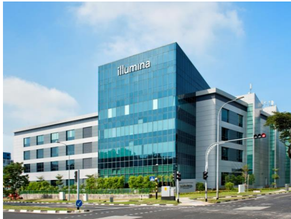
Repositioning of property into a modern and energy efficient hi-tech facility
