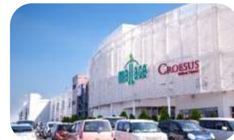
Mallage Shobu Suburban shopping centre in Kuki city, Saitama Pref.
