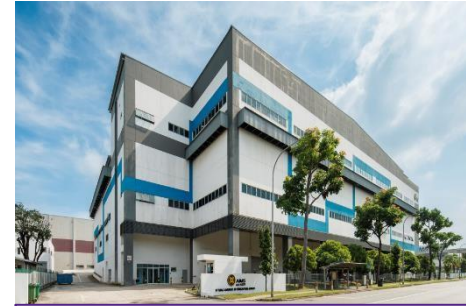
8 Tuas Avenue 20, Singapore
