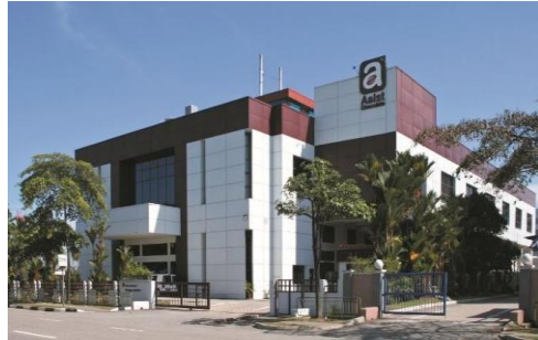
26 Tuas Avenue 7, Singapore
