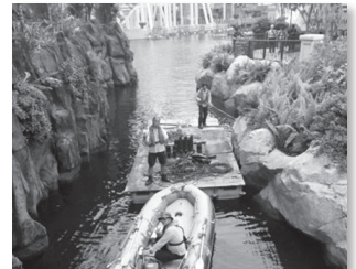
Positioning of floating platform
