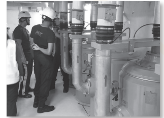
Inspection of Gas Filters
