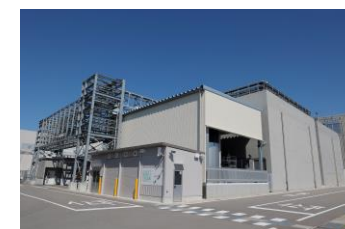
Facilities to treat liquid waste
