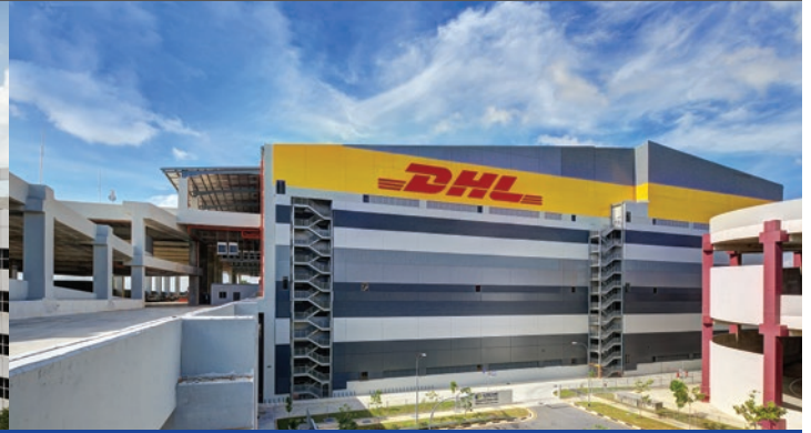
DHL Supply Chain Advanced Regional Centre 1 Greenwich Drive, Singapore
