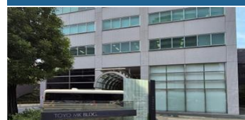
Toyo MK Fuso Building
