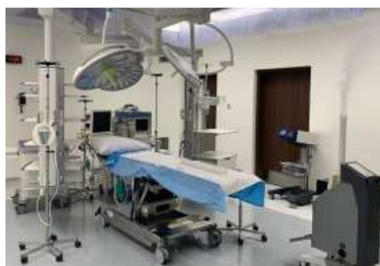
Figure 1: An example of a disinfecting device (bottom right corner) in an operation theatre.
