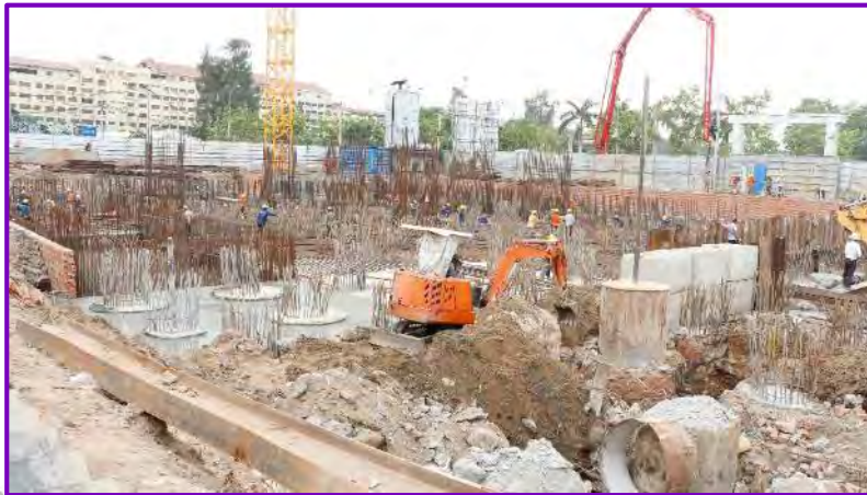
Construction Update as of April'15
