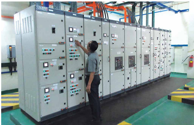
Air-conditioning chiller systems
