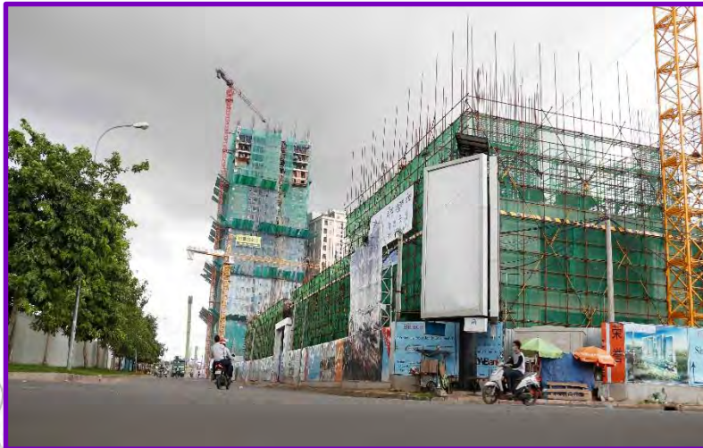
Construction progress as of Sep'15
