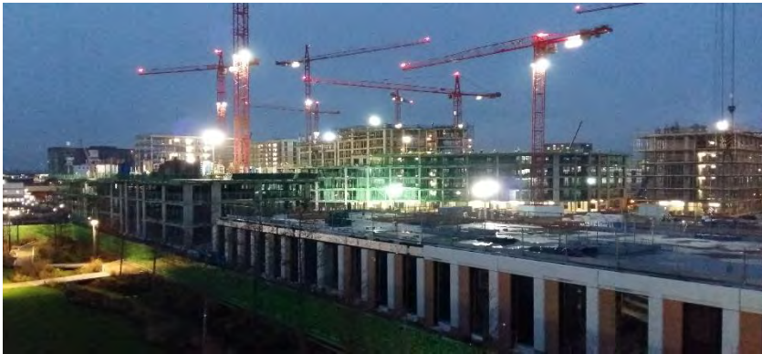
Construction progress as at 14 Dec 2015
