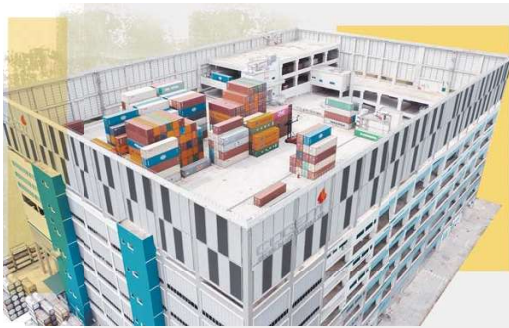
Cogent Jurong Island Logistics Hub (Phase 1)
