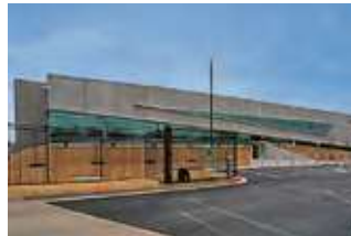
34 4121 & 4114 Perimeter Center Place, Oklahoma City
