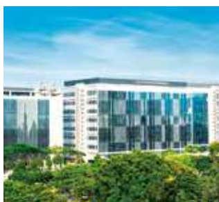
5 Mapletree Hi-Tech Park @ Kallang Way
