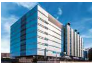
61 Osaka Data Centre
