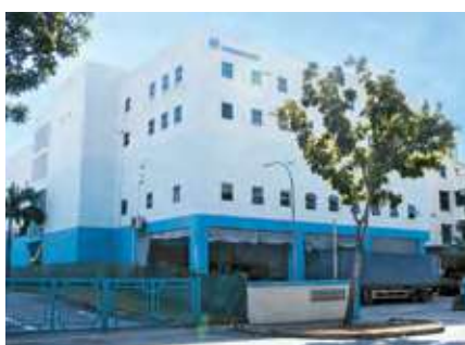
1 2A Changi North Street 2
