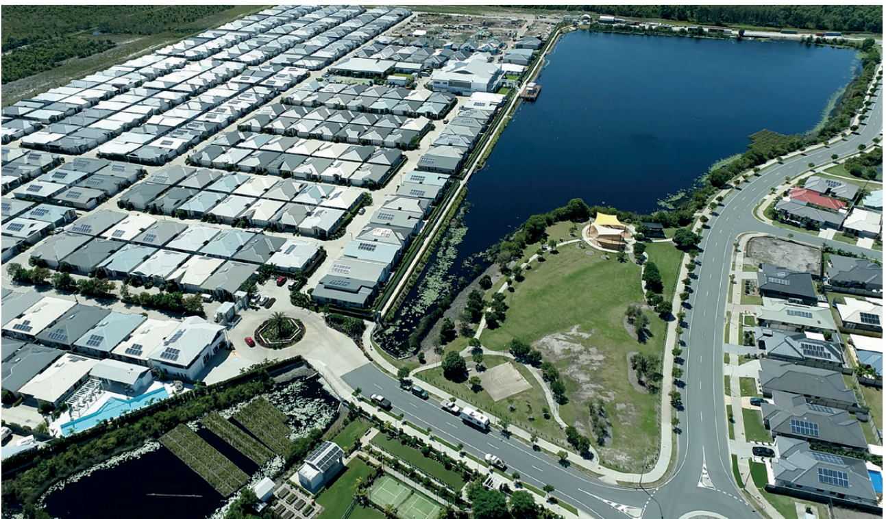
GEMLIFE BRIBIE ISLAND – HOUSES FITTED WITH SOLAR PANEL
