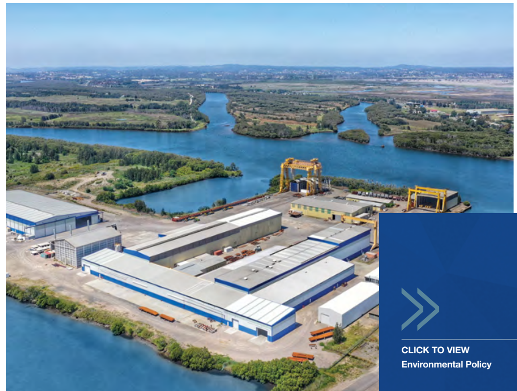
Right: Civmec's Tomago facility
