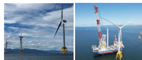
Turbine Generator Installation
