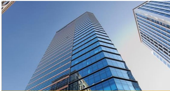
May 2019: Acquisition of T Tower in Seoul
