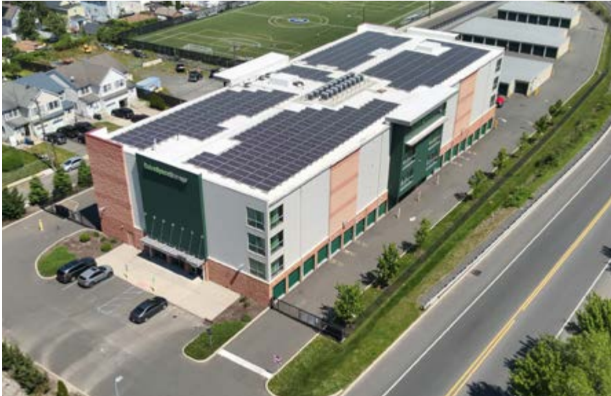
▲ Solar Panels on the rooftop of Carteret Self-Storage
