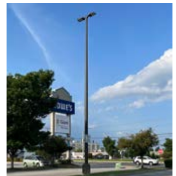
▲ LED Lighting Upgrade at Arundel Plaza: Enhancing Efficiency and Sustainability
