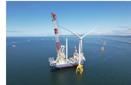
<Turbine Generator Installation>
