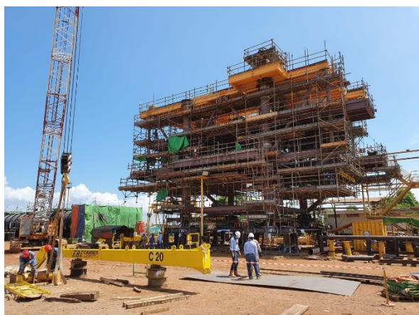
Apsara topside stacked decks with a width of 25.4 metres at the widest point and a structural weight of 210 MT
