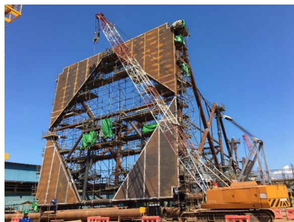
Mud mat installation of the Apsara mini-platform jacket, which has a vertical length of 76 metres and a structural weight of 577 metric tonnes
