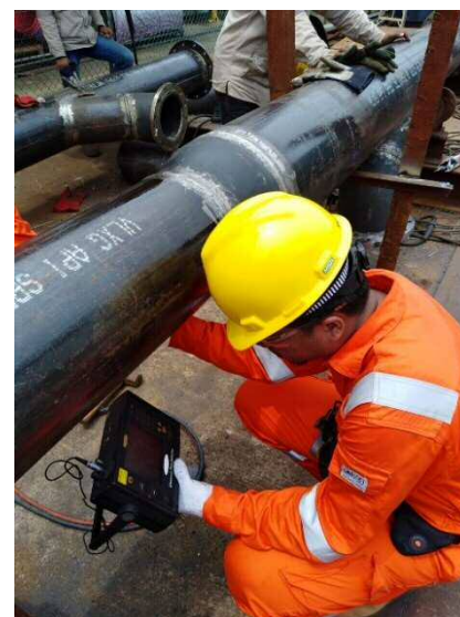
Above: Non-destructive testing conducts on fabricated pipe joints
