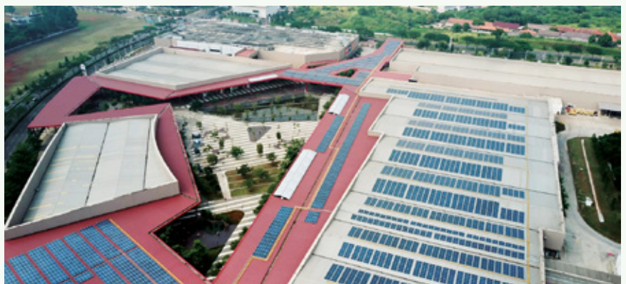
Solar panels on the roof of QBig BSD City
