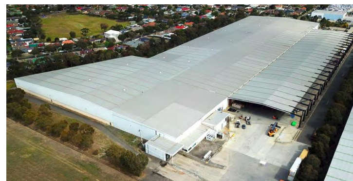
182-198 Maidstone St., Altona is located within a key established industrial precinct and is in close proximity to main roadways, the Port of Melbourne and Melbourne's central business district.
