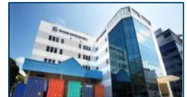
7 Cache Changi Districentre 2 3 Changi South Street 3
