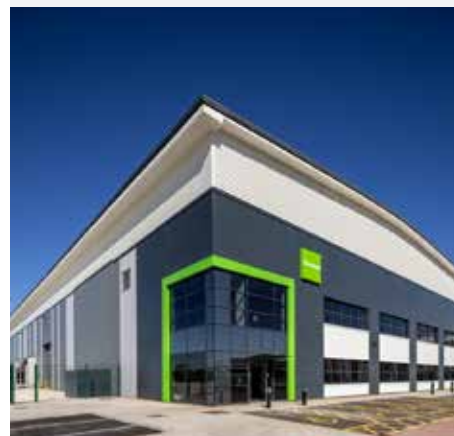
Crossways Commercial Park, Greater London, UK.
