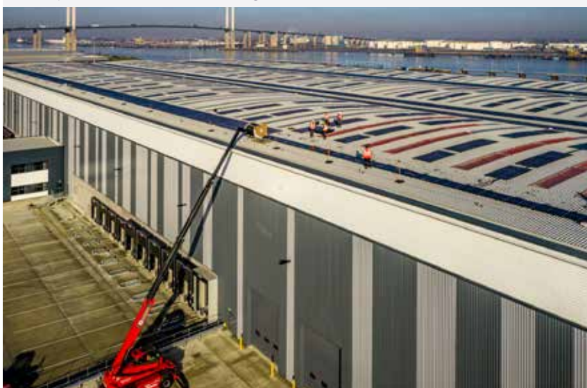
Crossways Commercial Park, London, United Kingdom.
