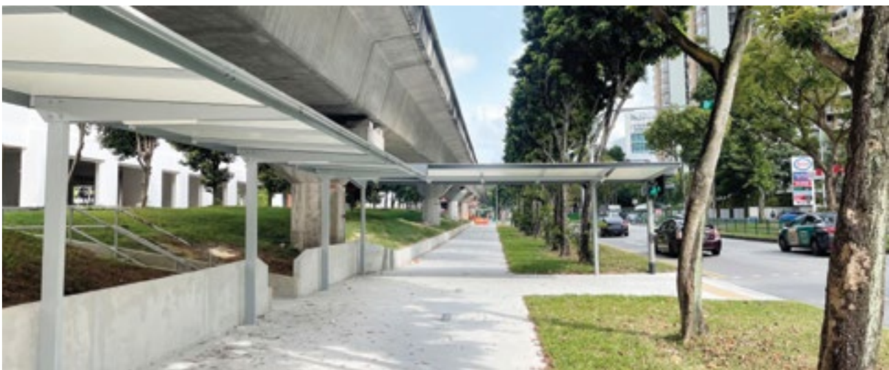
Under the Walk2Ride programme, OKP has completed the covered linkway at Keat Hong.
