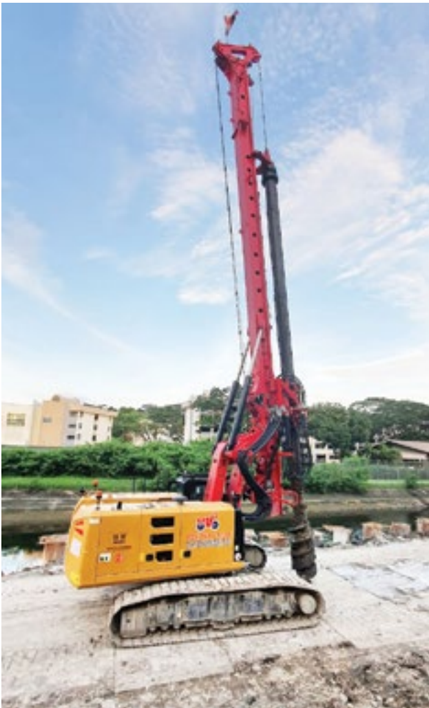
OKP purchased a rotary drilling rig for its construction works.
