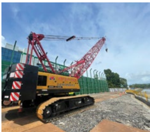
Newly purchased crawler crane to support OKP's construction projects.
