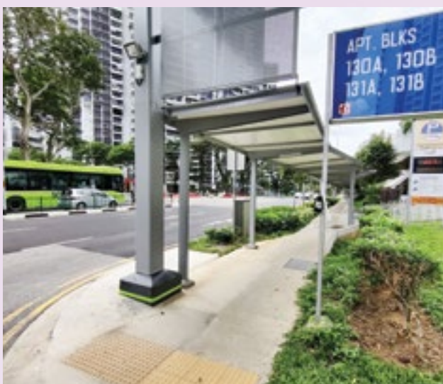
OKP is involved in the construction of covered linkways to Thomson East Coast Line Stage 1, 2 and 3 Stations.
