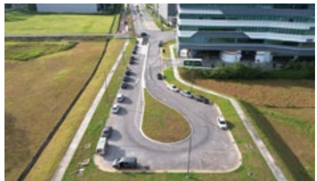
OKP has completed the construction of roads, drains and sewers at Portsdown Road.
