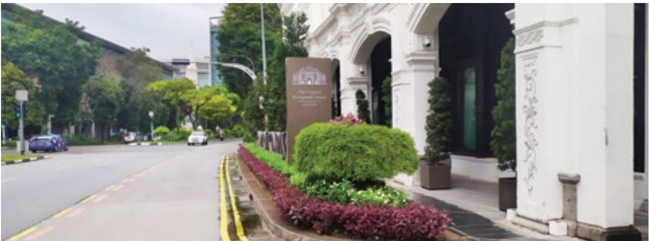
OKP has completed the improvement to roadside drains V contract C5 (Stamford Road, River Valley Road, Upper Thomson Road and Burghley Drive).
