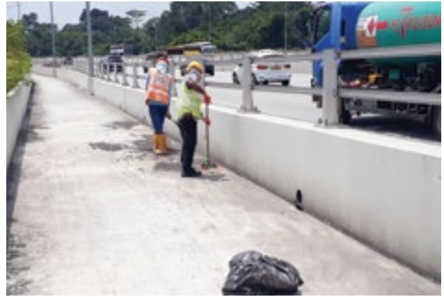
OKP has completed maintenance works at various locations.
