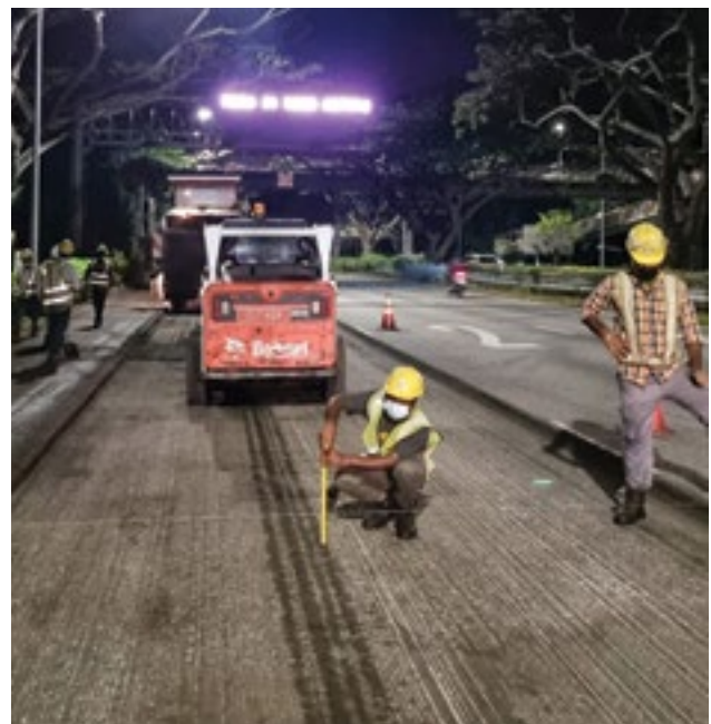
Road maintenance contract for Expressway is an ongoing project by OKP.
