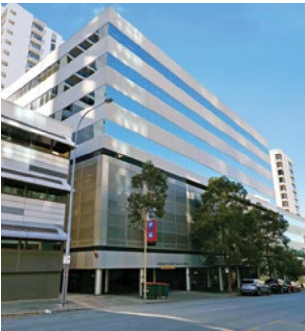
Exterior view of 6-8 Bennett Street in East Perth, Western Australia.
