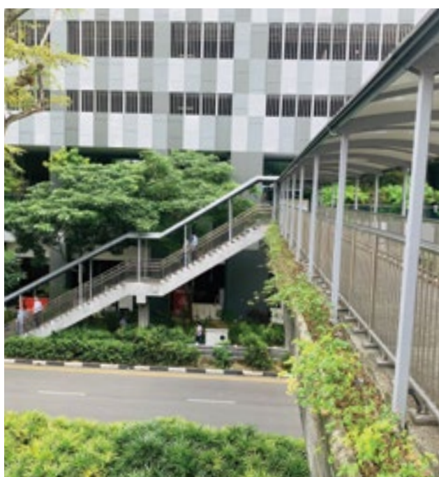
Under the Walk2Ride programme, OKP has completed the covered linkway at Nicoll Highway.
