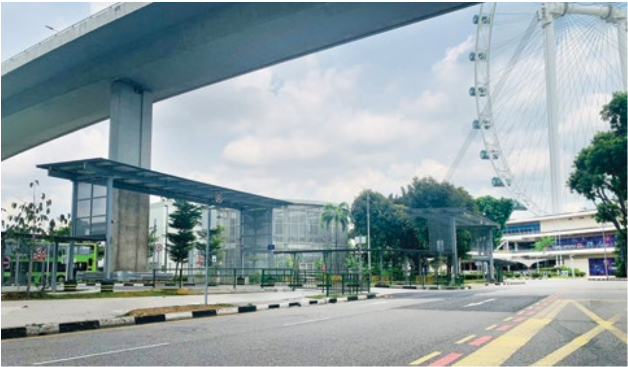
Under the Walk2Ride programme, OKP has completed the covered linkway at Promenade Station.
