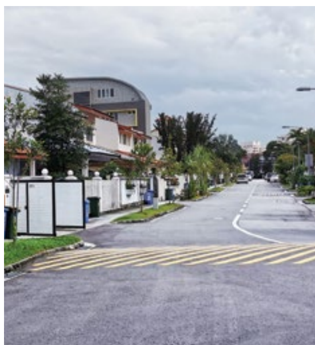
OKP is involved in the improvement to roadside drains V Contract E5 (Yishun Avenue 1/6, Jalan Kembangan, Pasir Ris Estate and Hai Sing Estate areas).
