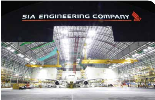
Hangar bay lights (LED)
