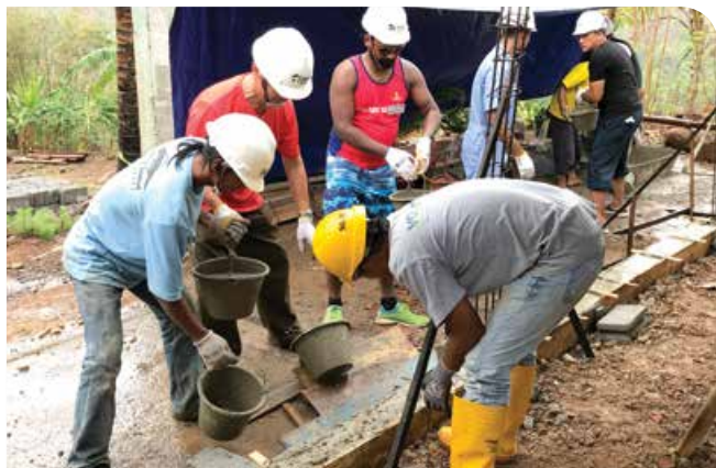
House-building in Yogyakarta, Indonesia
