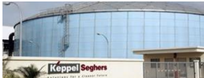
Keppel Seghers Ulu Pandan NEWater Plant
