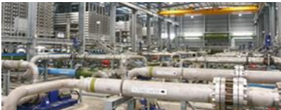
SingSpring Desalination Plant
