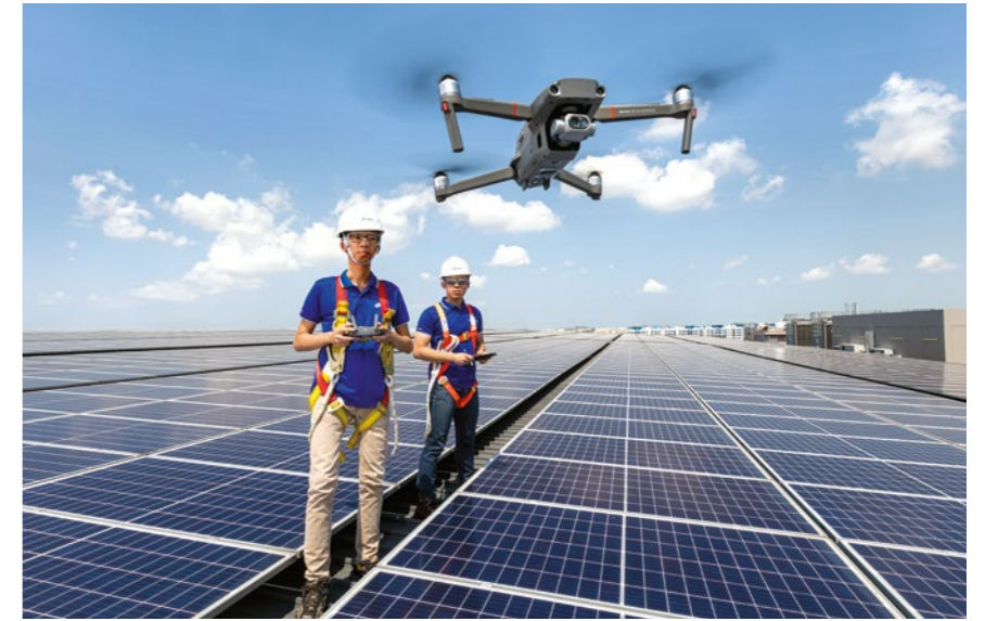
Sembcorp is one of Singapore's largest solar players with an additional 63MWp of solar capacity and 14 new commercial customers secured in 2019
