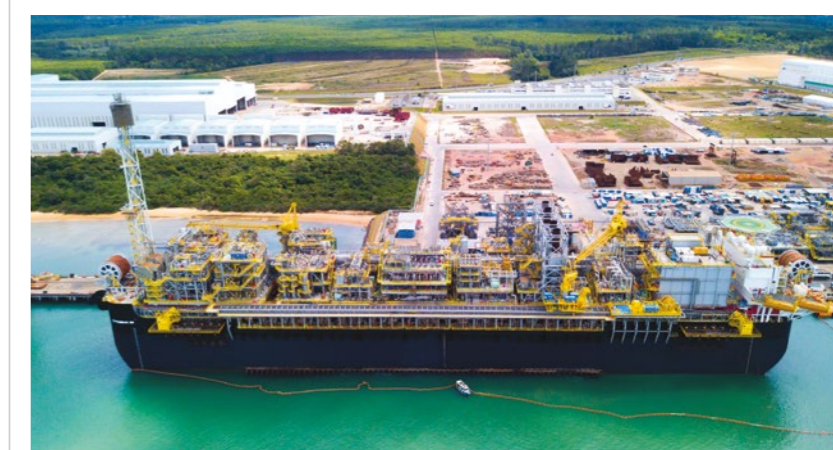
Topside modules construction and integration for the FPSO P-68 delivered to Petrobras, a testament to Estaleiro Jurong Aracruz's engineering, procurement, construction and commissioning capabilities
