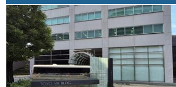
Toyo MK Fuso Building
