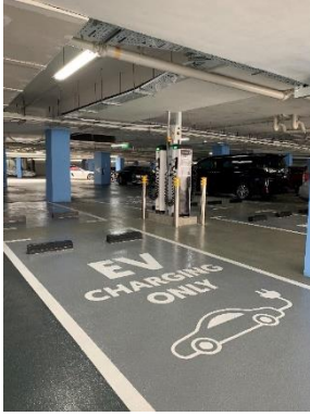
Electric vehicle charging stations at the Marina
