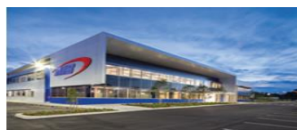
Martin Brower Facility, New South Wales, Australia
