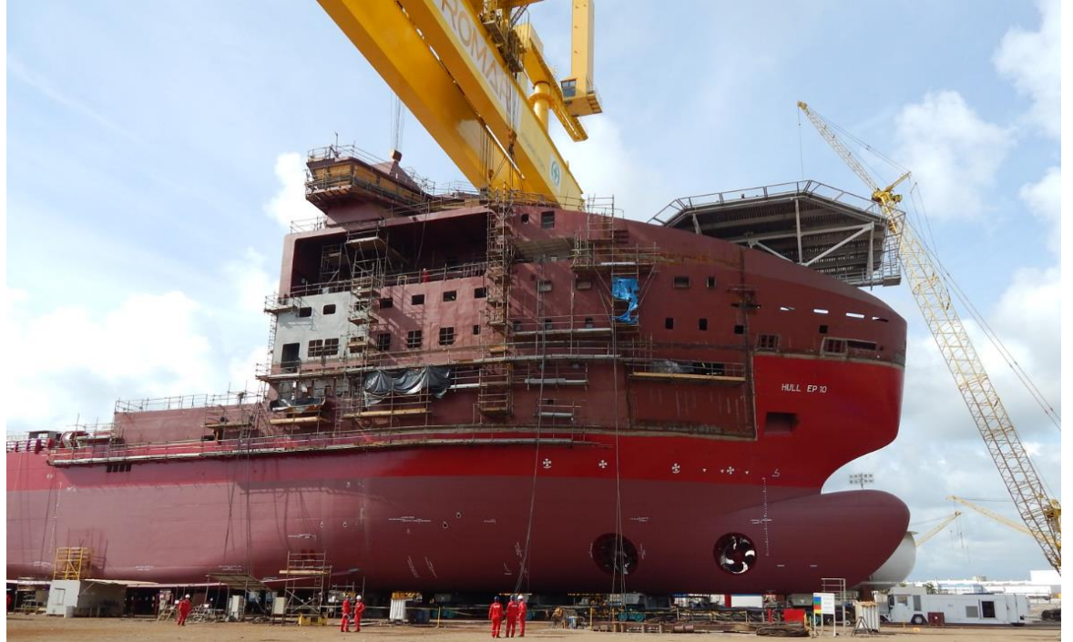
Vard Promar – PLSV for Dofcon Navegação under construction
