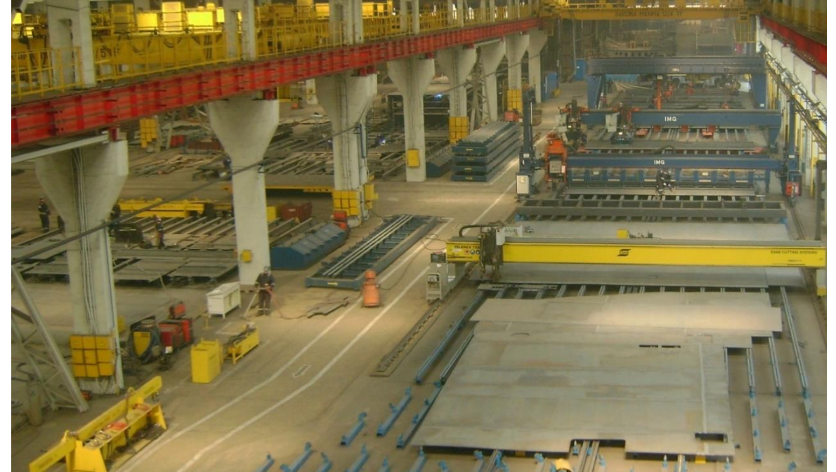
Vard Tulcea – view of the fabrication hall
