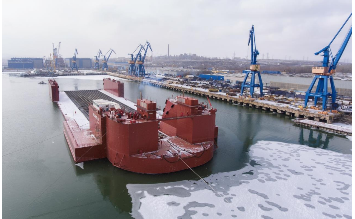
Vard Tulcea – enlarged launching barge Atlante II
